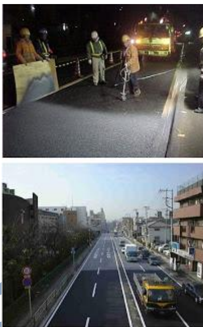
Fig 2.7. Using TiO 2 photocatalytic material as coating on roadway for pollution reduction: left; right – finished road showing a lighter colour (From Construction and Building Materials , 25 (2011), 588 )
