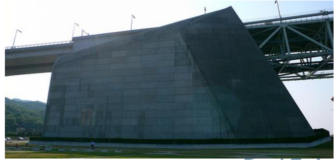
Anchorage of akashikaikyo bridge.
