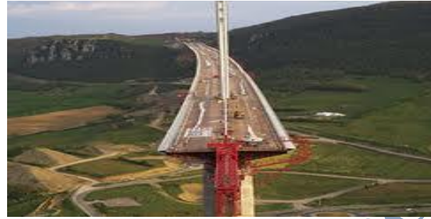
DECK BEING PUT IN PLACE
