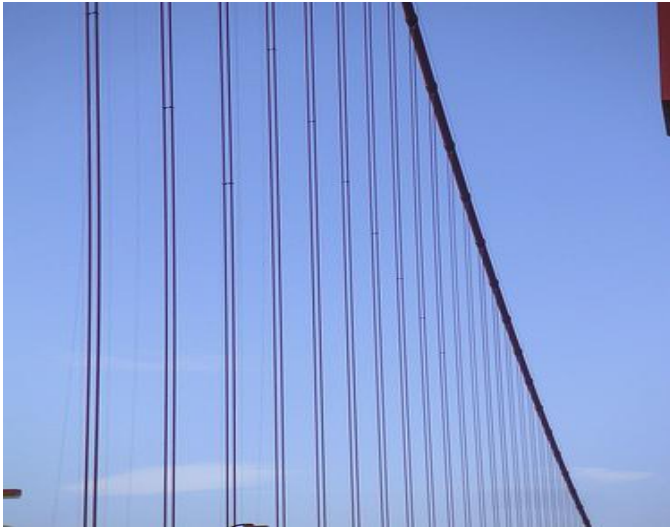
MASTER CABLE AND SUSPENDED CABLE IN PLACE
