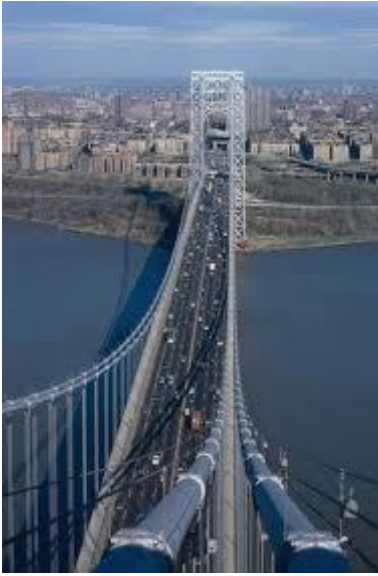
Completed deck work
