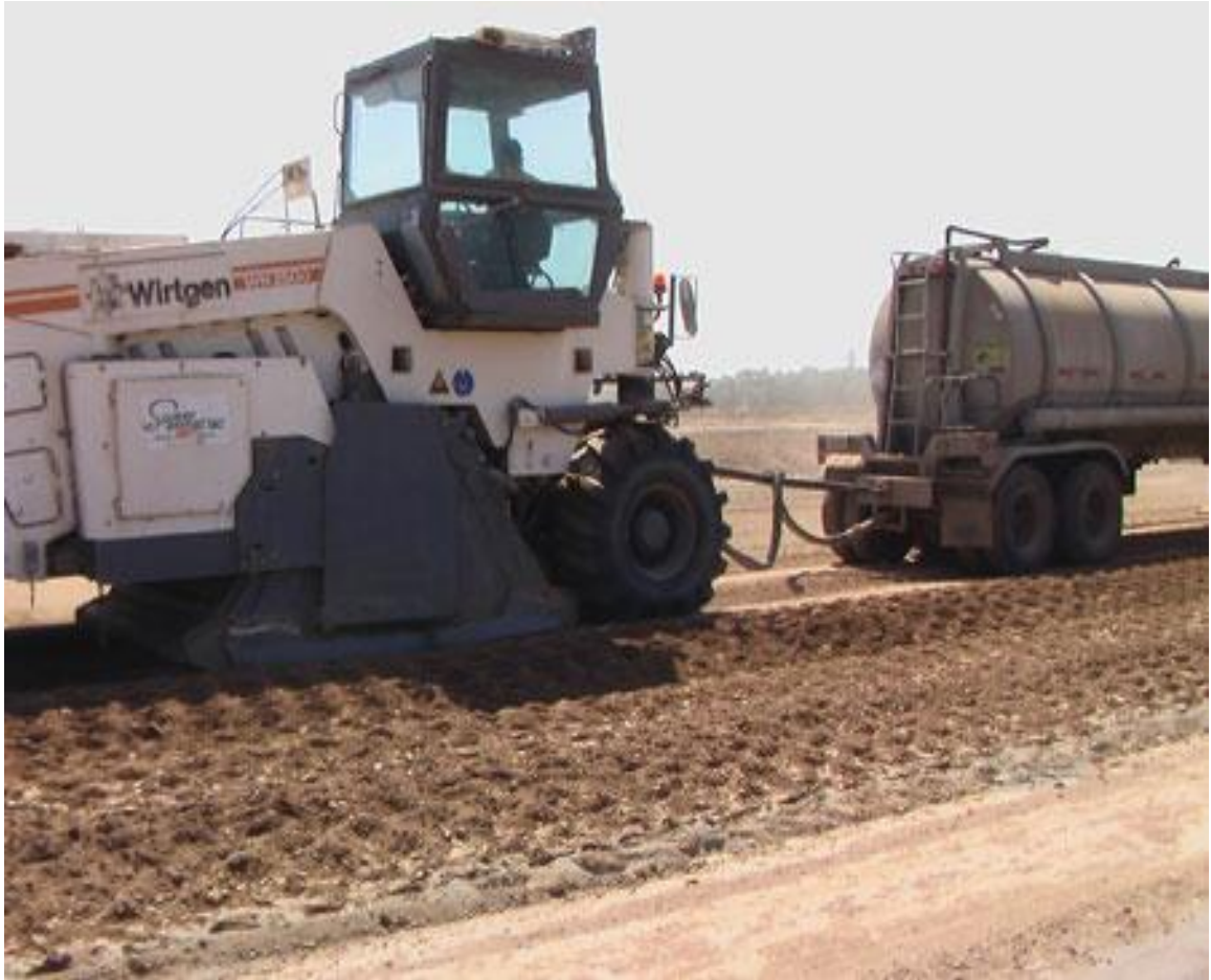
FIG.2. Mixing of soil-cement for sub-grade stabilization
