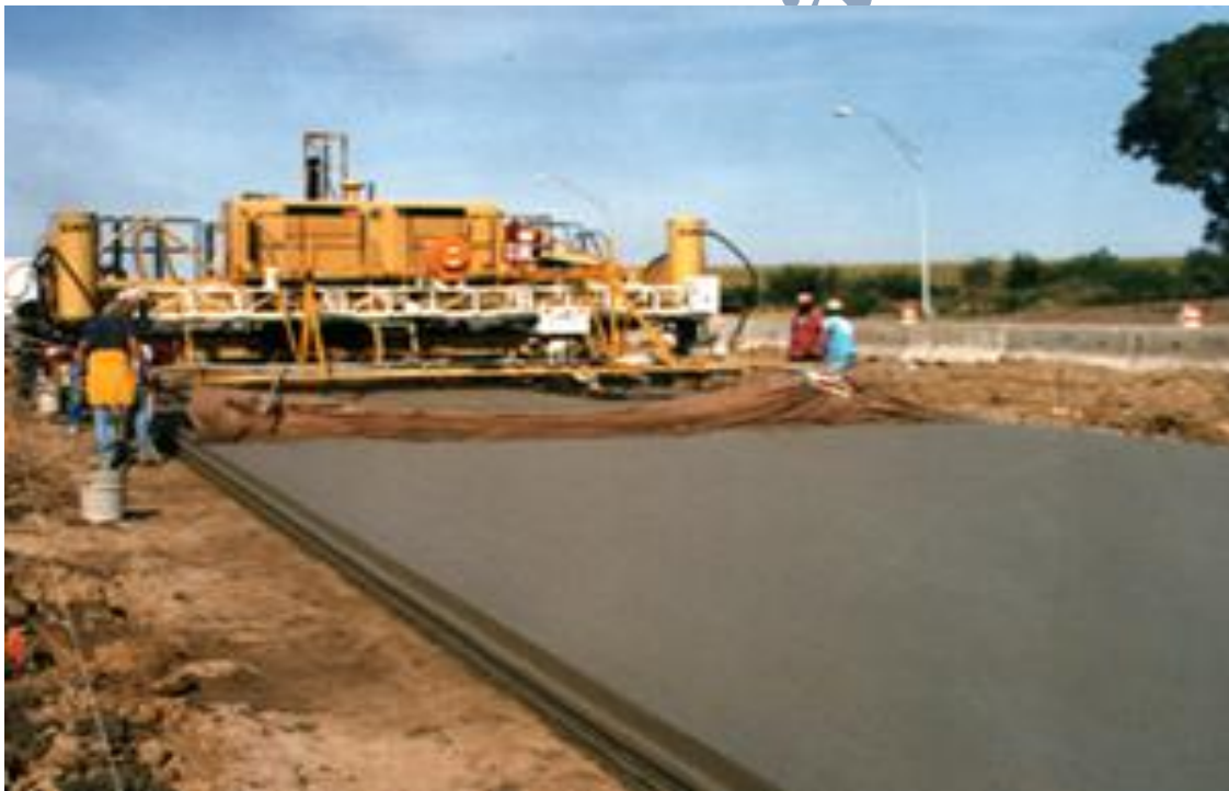
FIG.4.FLY ASH IN CONCRETE
