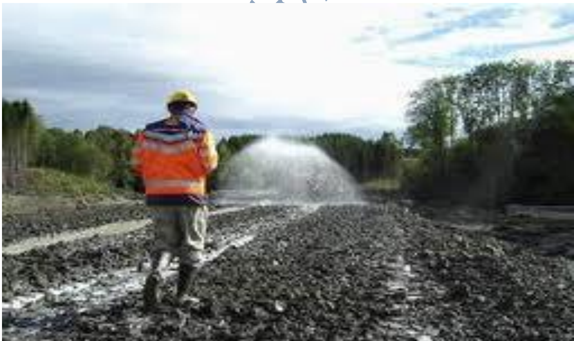
FIG.3. Soil stabilization with bitumen
