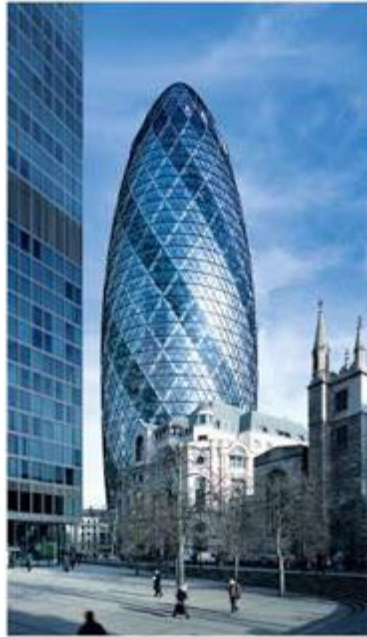
Figure 14: Swiss Re Building, London
