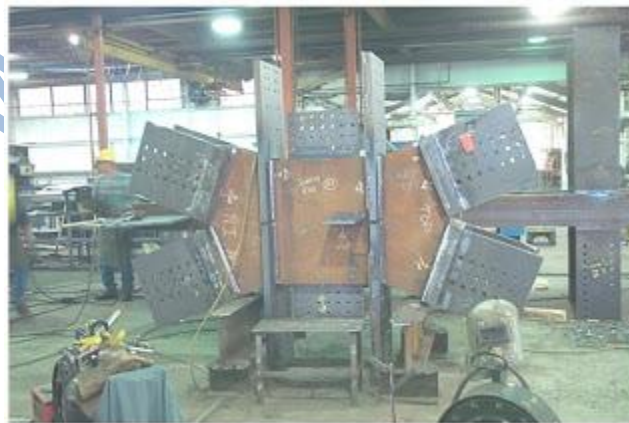
Figure 11: A Diagrid node after fabrication
