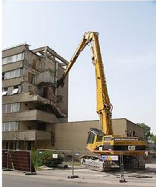
Fig 5. High reach excavator
