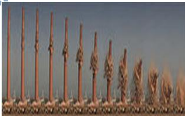
Fig 6. Demolition of a chimney in Germany (falling into footprint)
