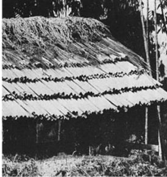
Fig 5(a) Double layers of bamboo shingles
