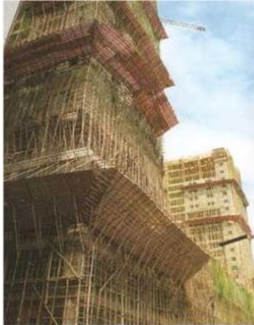
Fig 6 Bamboo canes used for scaffoldings
