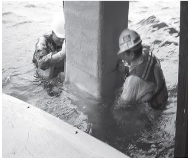
Fig. 2.9 Wrapping of FRP material around piles
