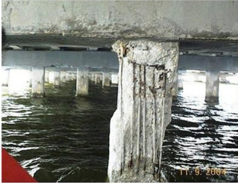
Impact damage that led to both cross-section loss and breakage of the spiral ties
