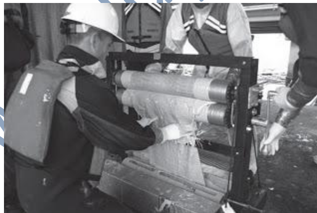
Fig. 2.10 On-site saturation, Friendship Trails Bridge, Tampa
