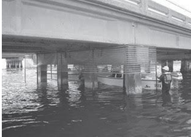
Fig 2.7 Mesh flooring around piles
